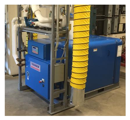
Together with our partner, Tecogen Incorporated, of Waltham, Massachusetts, TitanGen commissioned and constructed a 75 kW Tecogen CHP system for the purpose of creating domestic hot water, hydronic heating during the winter months and electricity all year-round. The end result for the customer was a truly cost-effect way to create the usable energy they
